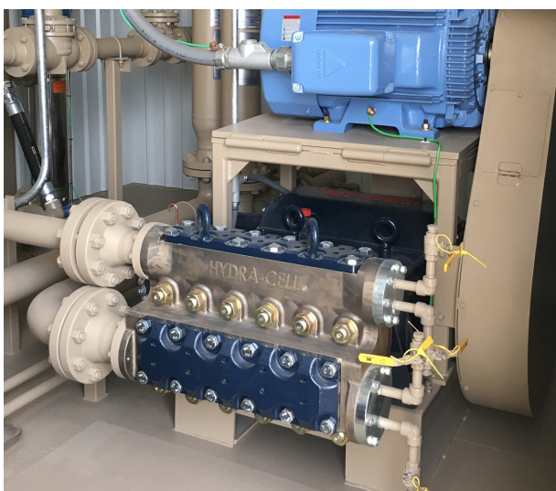
Figure 4. Hydra-Cell Q155 pump on transfer duty at a lease automatic custody unit.
