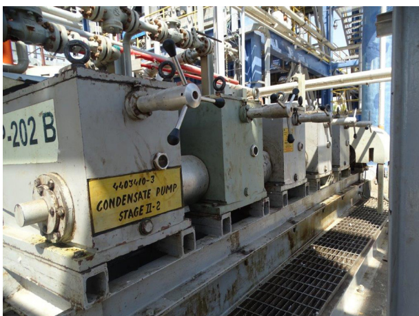
Figure 1. Pumps replaced: a battery of five linked traditional metering pumps on a condensate application (one diaphragm/head).
