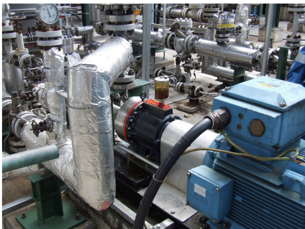
Figure 3. Pumping a hot water and chemicals mix to flush out main process pipes and minimise corrosion.
