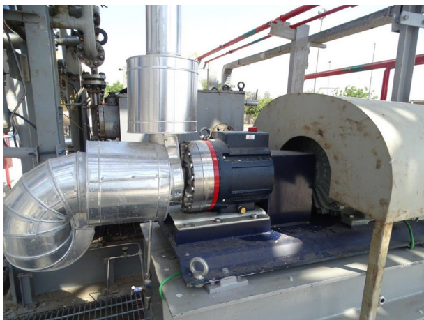
Figure 2. The replacement pump: a single Hydra-Cell pump on the same system to perform the work of the five linked traditional metering pumps.
