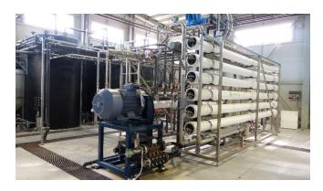
Wanner's Hydra-Cell pumps are running up to 10 m³/h @ 120 bar (1740 psi) at the two high pressure reverse osmosis systems and up to 15 m³/h @ 80 bar at the reverse osmosis stage 1.
