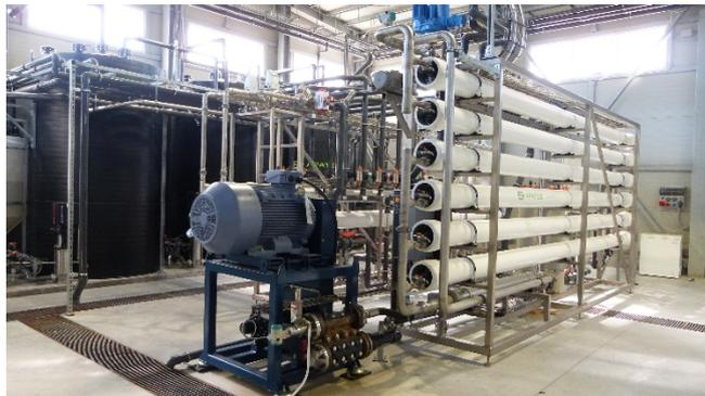
Wanner's Hydra-Cell pumps are running up to 10 m<sup>3</sup>/h @ 120 bar (1740 psi) at the two high pressure reverse osmosis systems and up to 15 m<sup>3</sup>/h @ 80 bar at the reverse osmosis stage 1.
