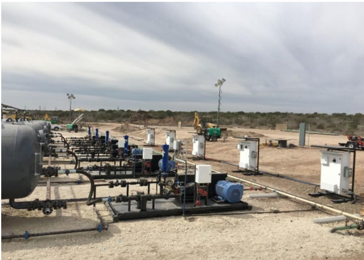
For over 40 years, Wanner has been designing, manufacturing and selling Hydra-Cell API 674, seal-less and packing-less positive displacement, hydraulically balanced diaphragm pumps for the oil and gas industry; a unique solution as a power fluid surface pump combined with downhole jet pump technology for a controllable and reliable production solution and optimisation.
