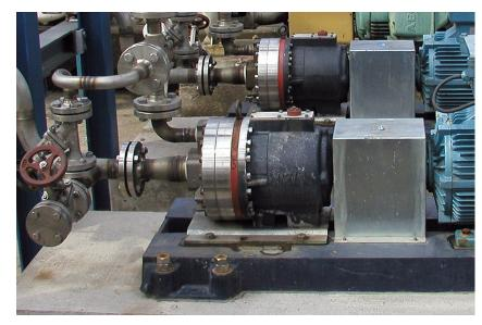
running against the shaft without cooling by liquid seepage causes overheating, seizure and catastrophic failure.
