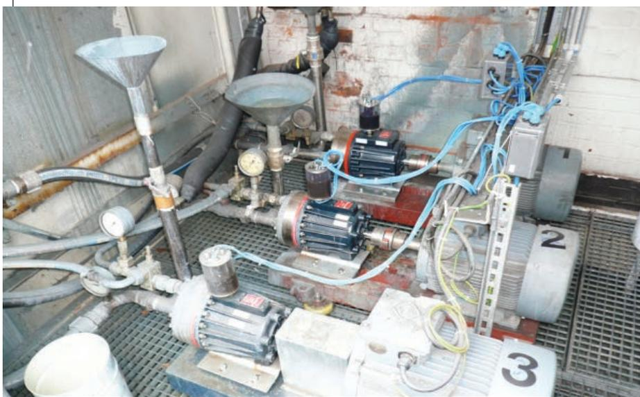
Seal-less Hydra-Cell G25 pumps replaced seal-reliant piston pumps handling recycled solvents on this mixing vessel cleaning system at a German paint manufacturer.
