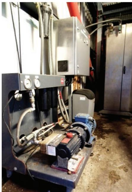
Pumping system with Hydra-Cell G03 serving humidifying nozzles. This pump replaced a 'high-maintenance' piston pump at the plant.
